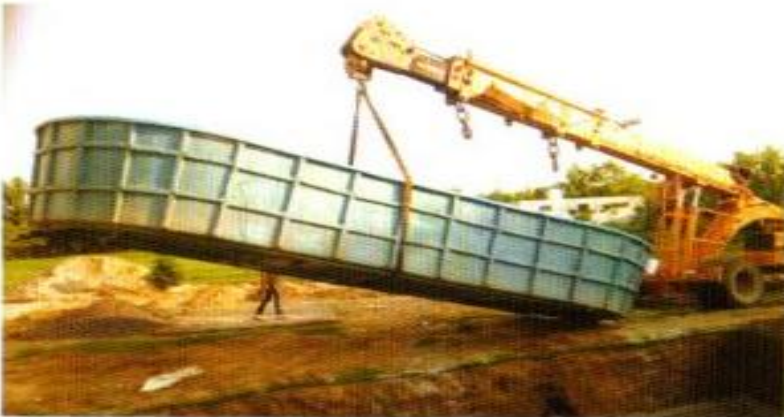
4. Lifting of swimming pool and placing on the prepared floor.
