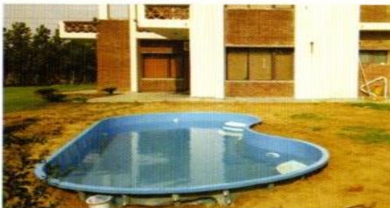
5. Filling water in pool and make deck area.
