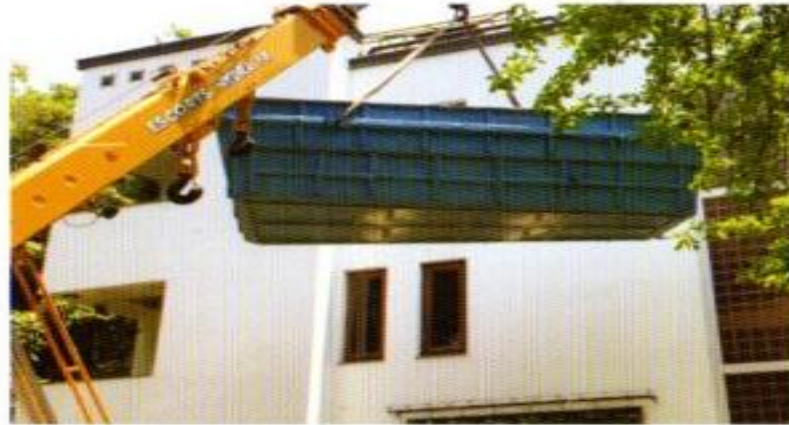
2. Placing the pool with the help of Crane at site.
