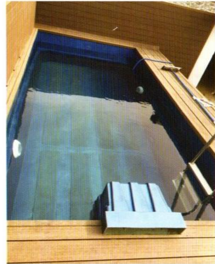
5. Filling the swimming pool and cover it to protect the water from Heat, Cold and Dust.
